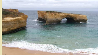
London Bridge after collapse.
