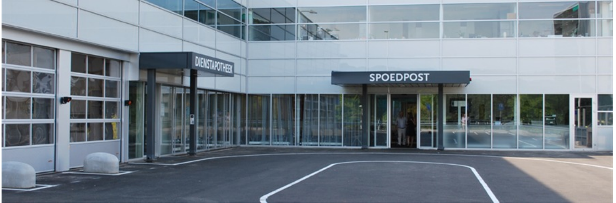
Emergency department (ED) of Catherina Hospital Eindhoven
